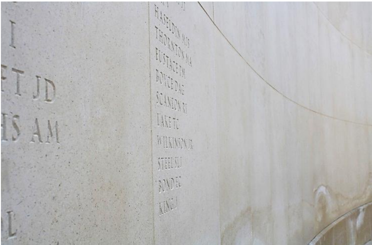
Figure 6: The curved engraved wall, also showing the large blank space awaiting new names Photograph: Callum Hogg, March 2013
