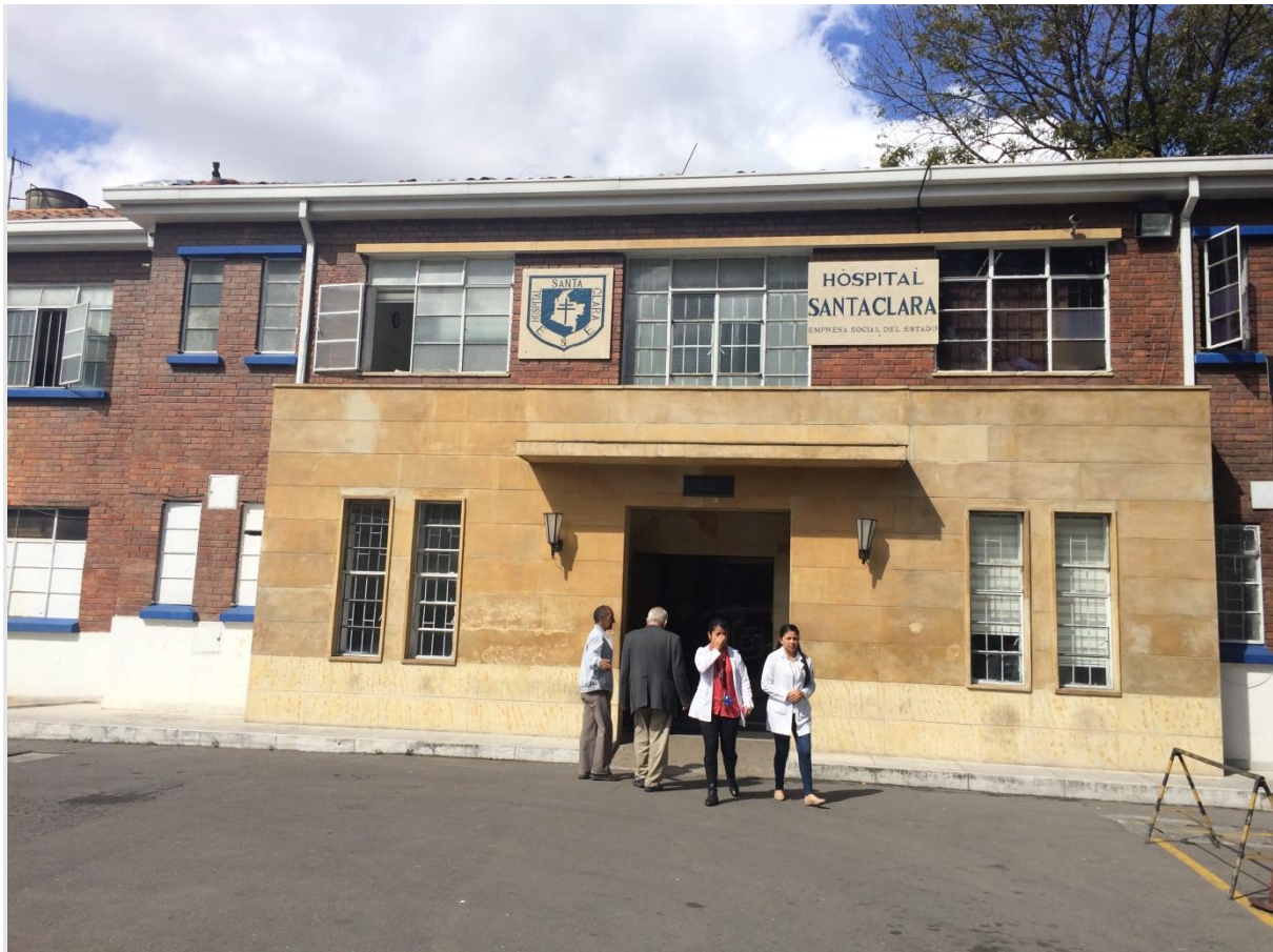
Figure 5. Santa Clara Hospital
